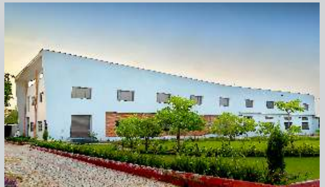
Tempsens Instruments U# II - MI Cable Plant
