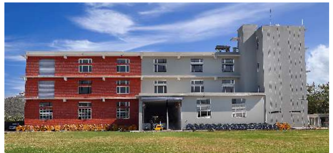
Tempsens Instruments U# IV Cable Plant
