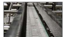
Conveyer Belt Monitoring
